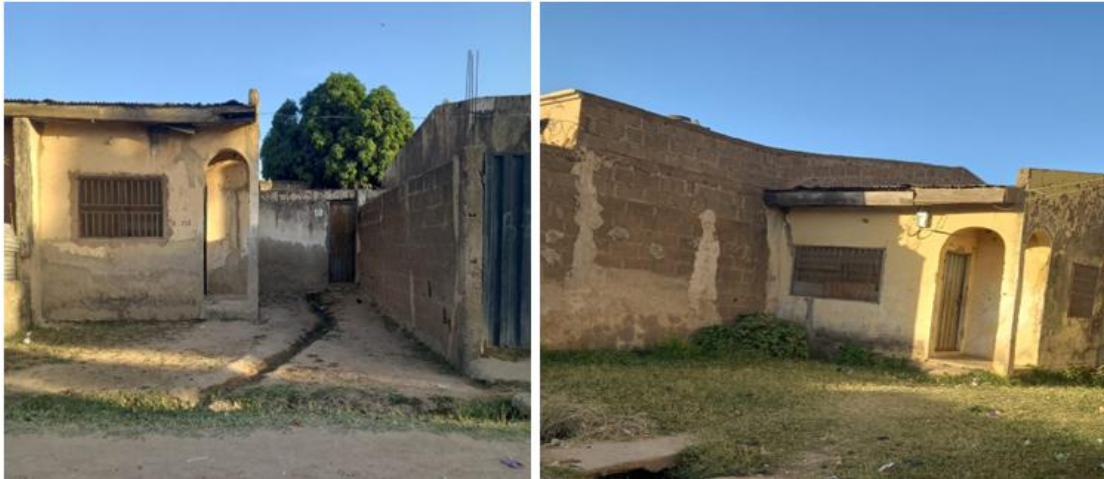
Figure 12: Existing low-cost housing at Danladi Nasidi.
