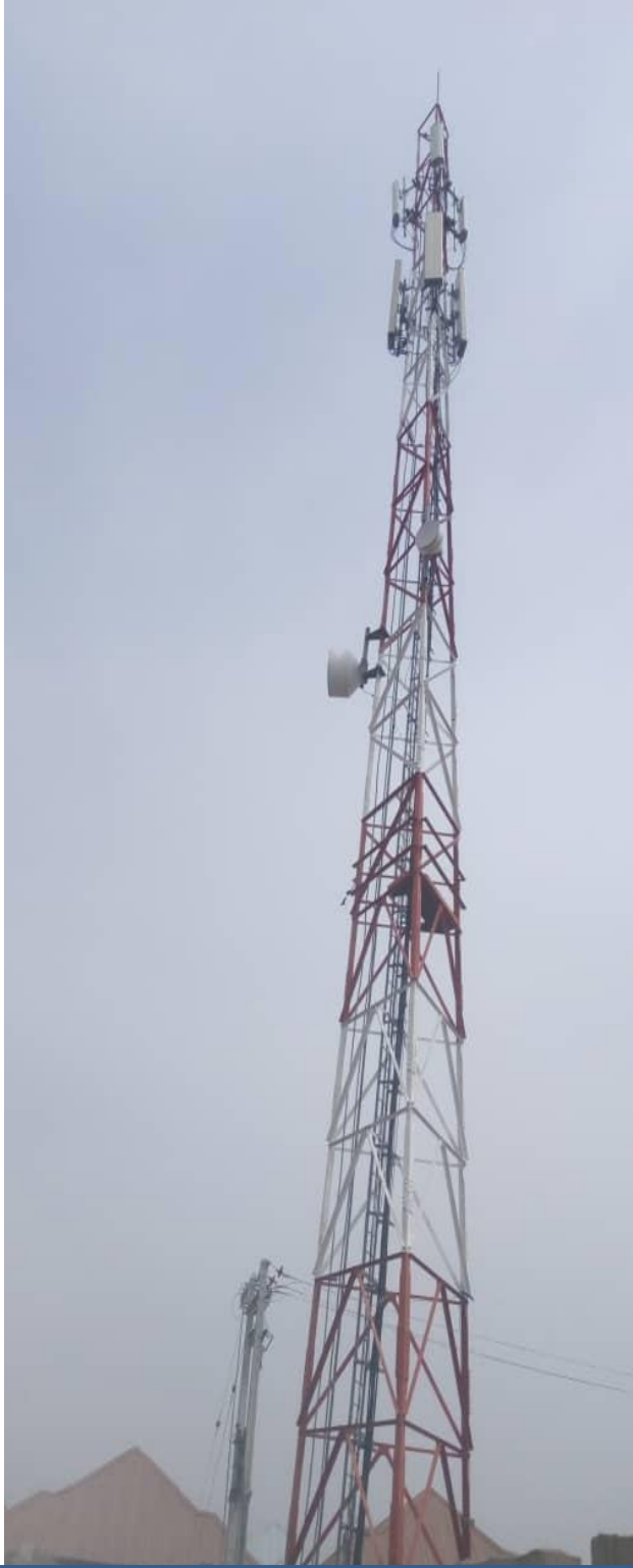
Plate III: Two RF and six MW antennas
