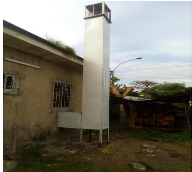
**Figure 1:** HDEC integrated into an office building
